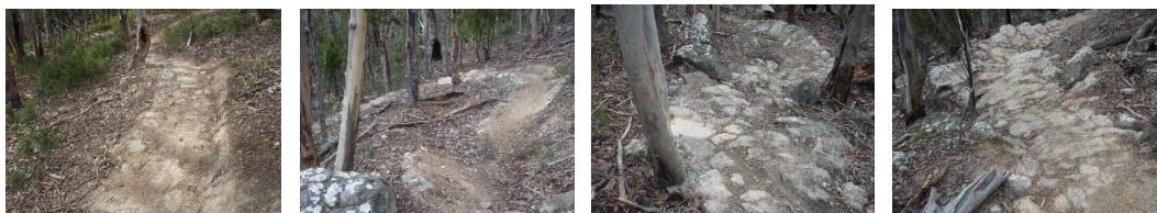
Tip Top Track – paving work
